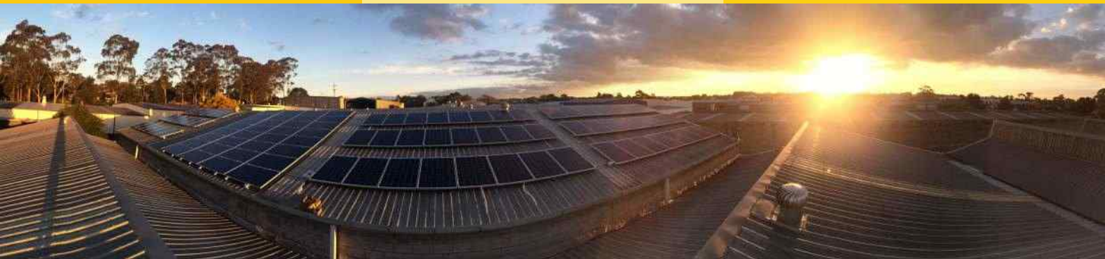
Girraween NSW 25 kW system June 2014
